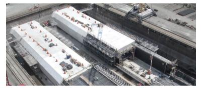
The chosen construction method for the new tunnel was using large float-in concrete sections, immersed into a dredge trench, and connected. The immersed tunnel option
